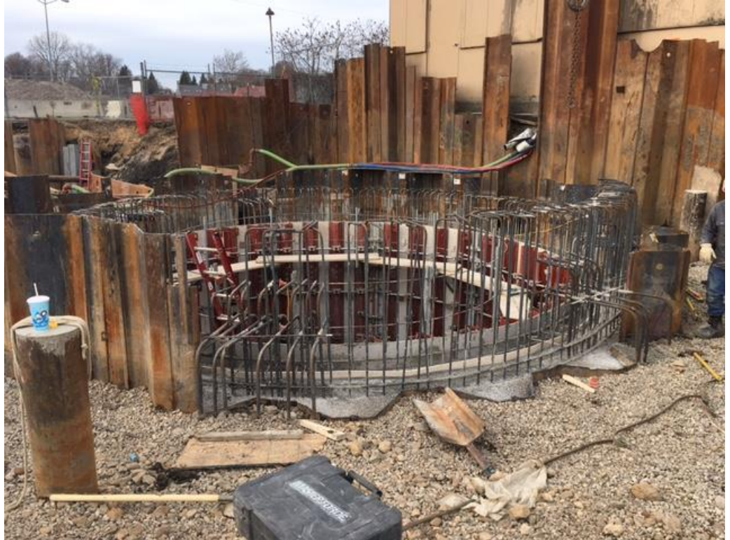
Wet Well Progress.
